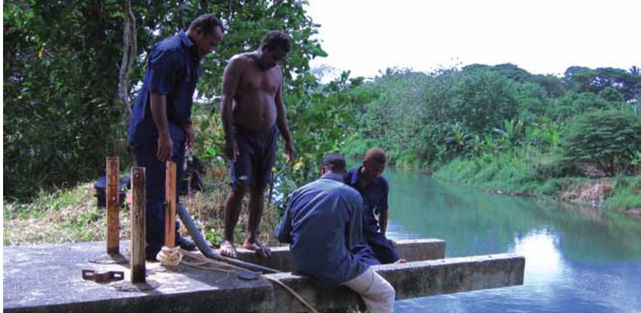
Site refurbishment, Lungga River, Guadalcanal
