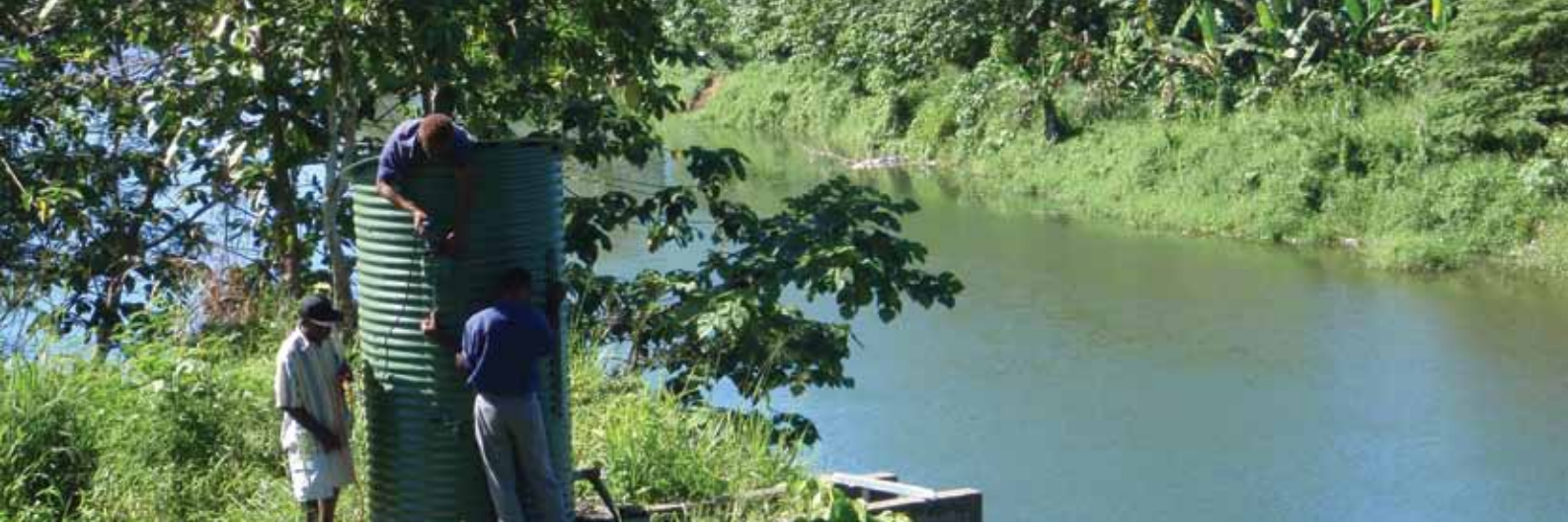
Lungga River, construction of security housing
